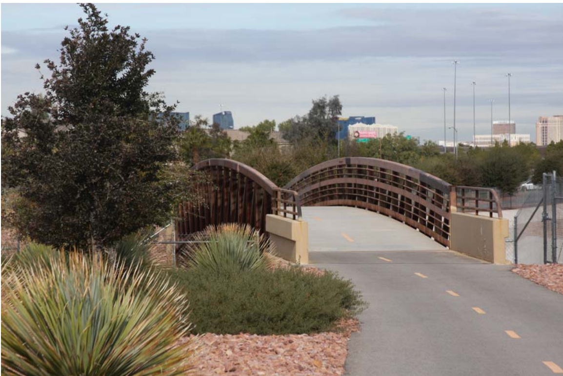
I-215 East Beltway Trail – North of Windmill
