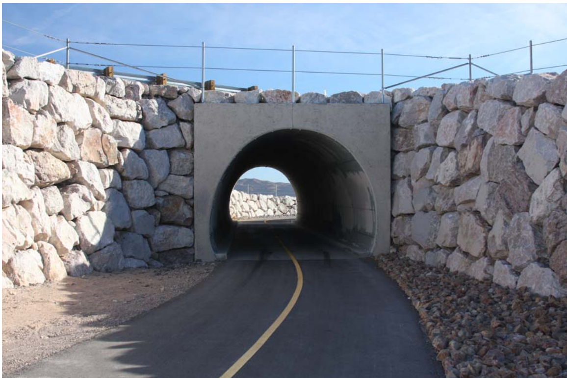
Flamingo Arroyo Trail Wayside – Underpass Beneath Hollywood
