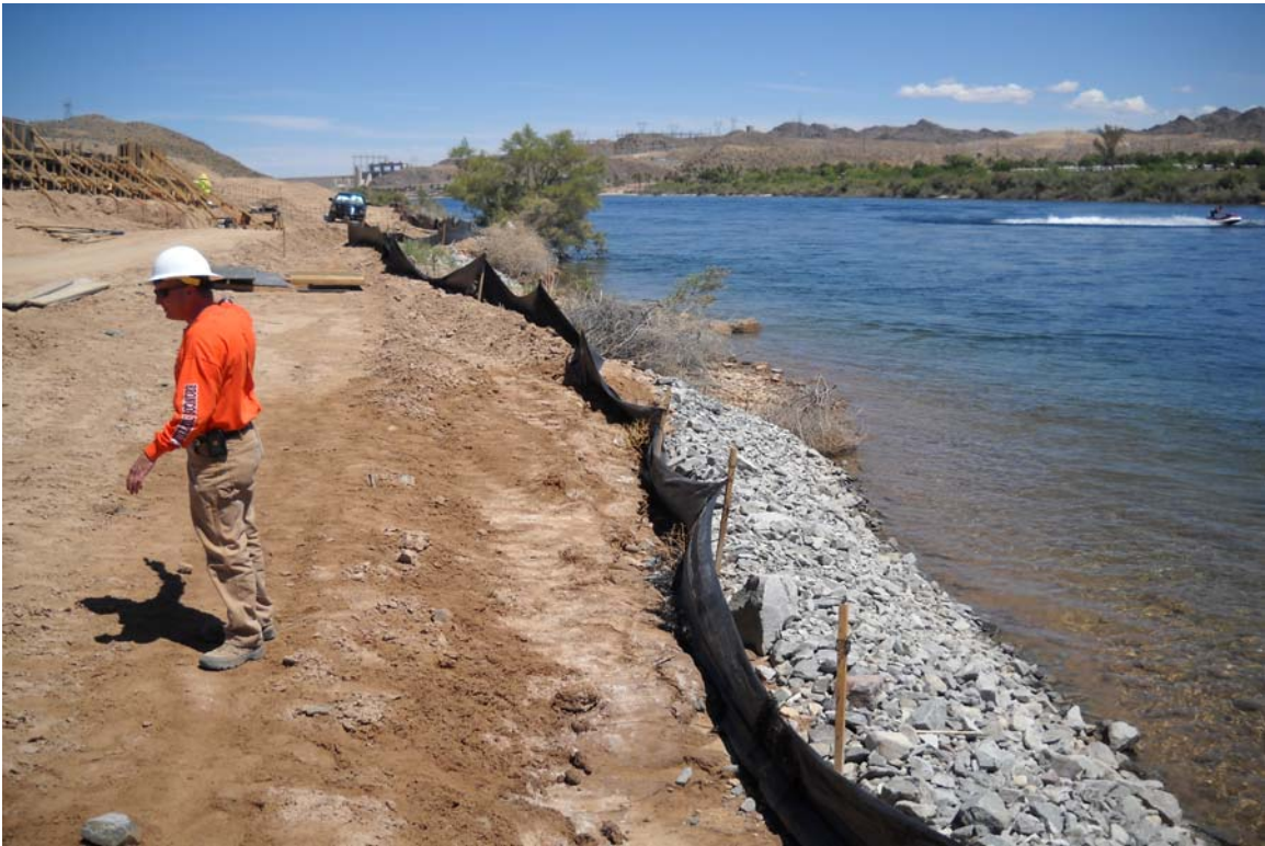
Trail Construction Along the Colorado River
