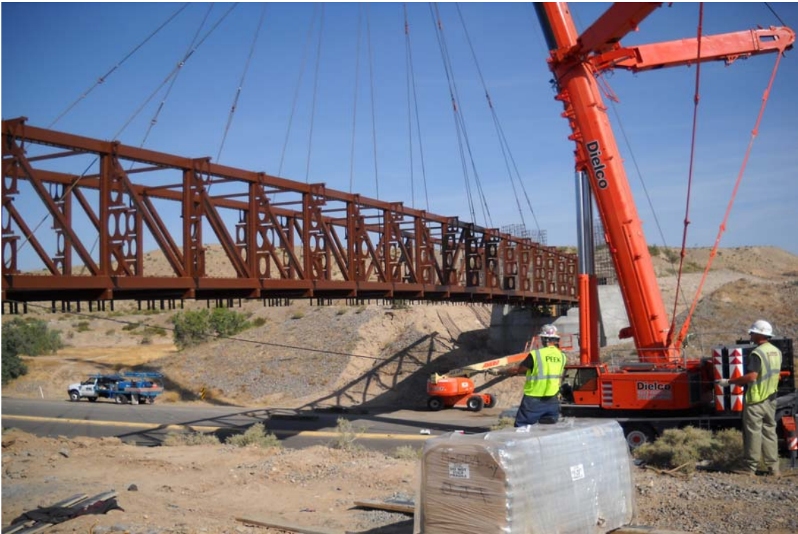
Carefully Setting The Bridge On Massive Supports
