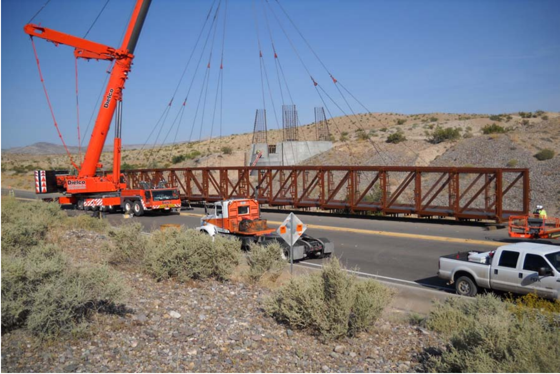
Lifting Huge Pedestrian Bridge That Will Span Nevada SR-163
