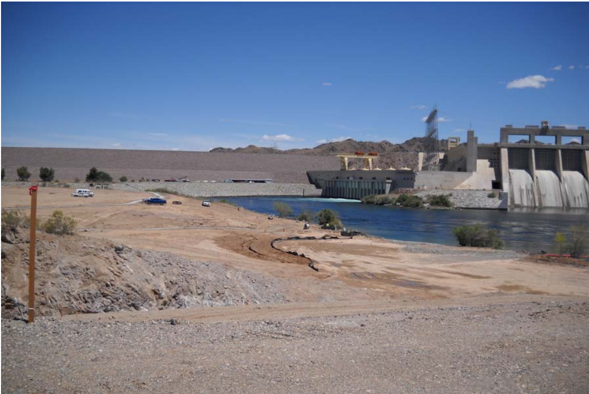
Construction of Day Use and Camping Area By Davis Dam
