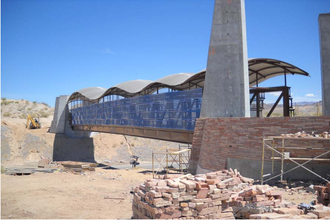
Bridge Being Finished With Roof and Side Enhancements
