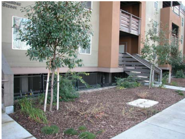
Example of inappropriate method of screening views into the podium parking level (prohibited)
