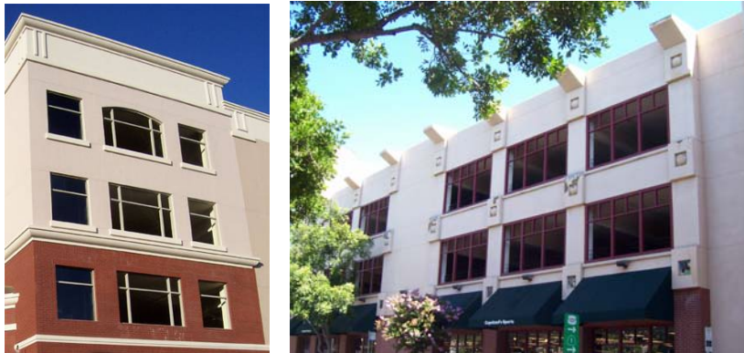
Examples of appropriately designed parking structure facades
