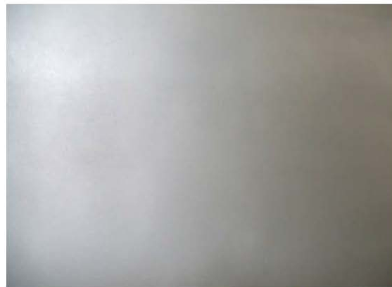
Figure 6: Redecorate Repaired Area
