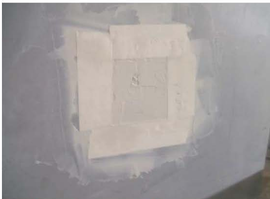
Figure 5: Tape and Finish Patched Area
