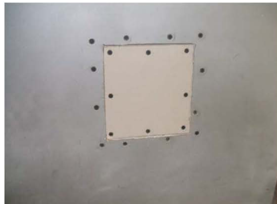
Figure 4: Apply Gypsum Panel Patch
