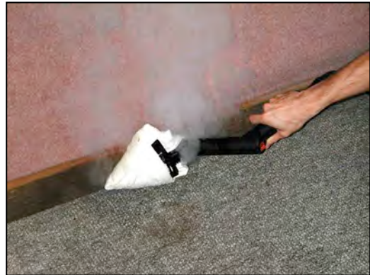
Steam cleaning the baseboard. Note that the wand is covered with a terry wash cloth to increase and retain heat. Photo by R. Cooper.
