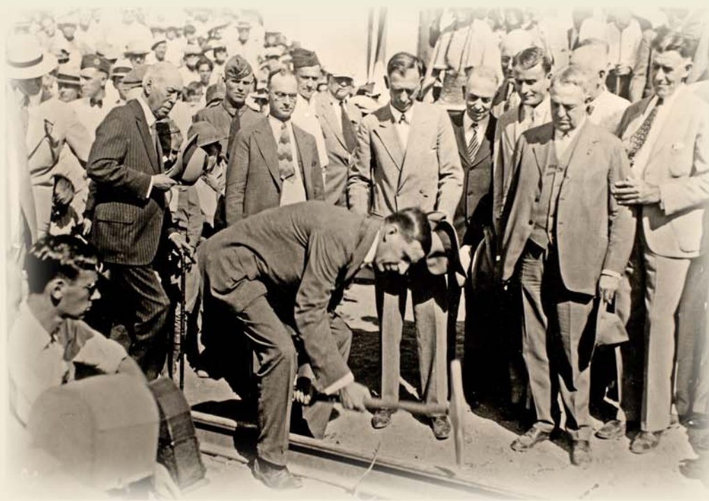
Secretary of Interior Ray Lyman Wilbur drives home the silver spike to begin construction of the Boulder Branch Railroad to Boulder City townsite, September 17, 1930. - Special Collections, Lied Library, UNLV
