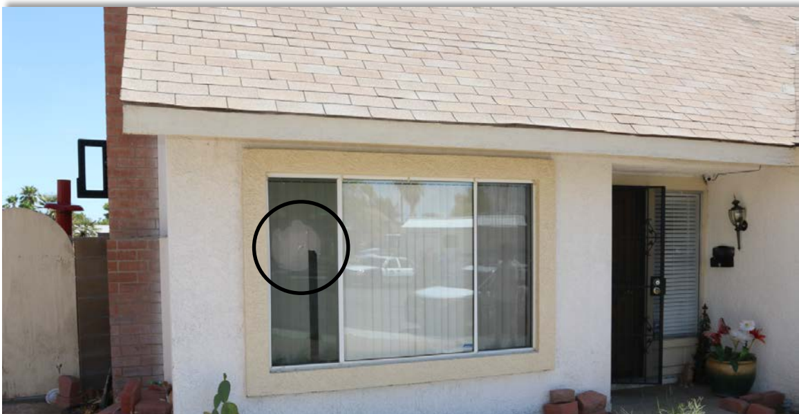
Figure 2. The ball hitch traveled through the window closest to 6990 Berkshire Place, the neighboring house.
